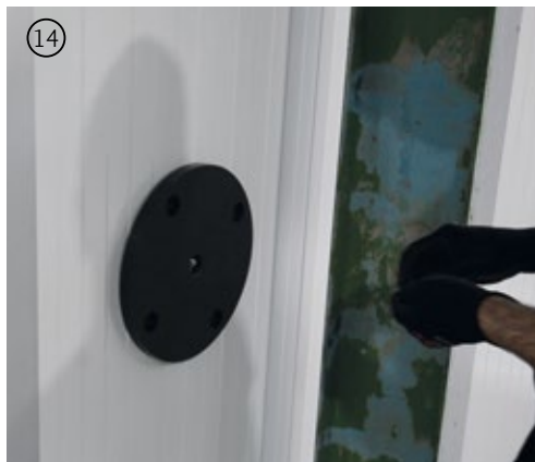
Colocar peana sobre pared/panel Place base on wall/panel
