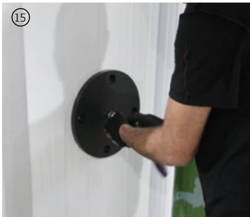
Enrosca tuerca a varilla Screw nut to rod
